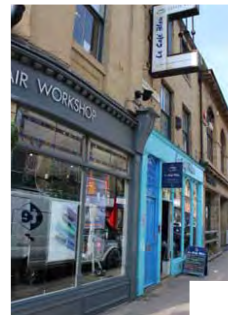
North Parade shopfronts
