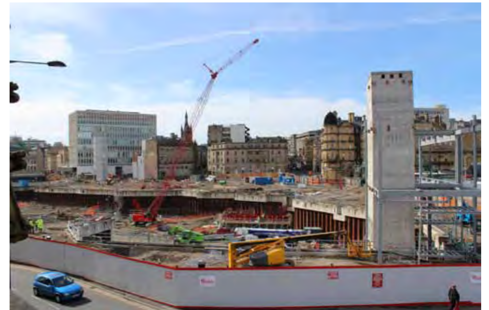
Westfield Broadway under construction
