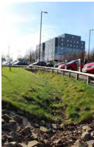
SUDs swales on Longside Lane
