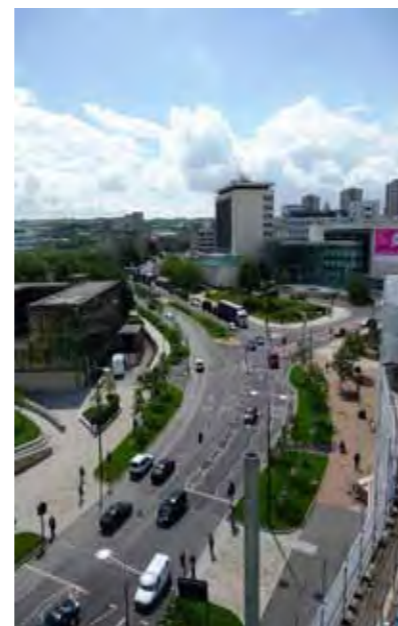
Prince's Way refurbishment
